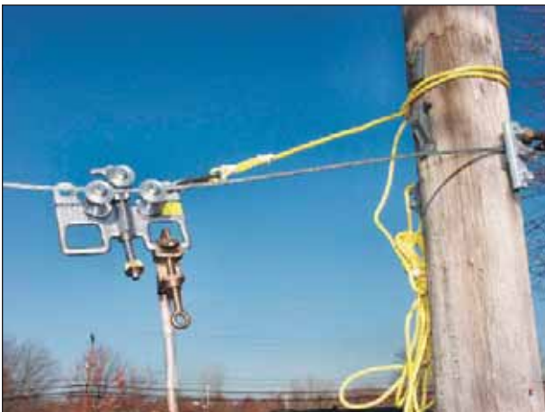
Grounding roller on messenger strand
