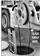
the pulling tension must be limited by means of a break-away swivel or by limiting the hydraulic system pressure to achieve a maximum allowable torque.
