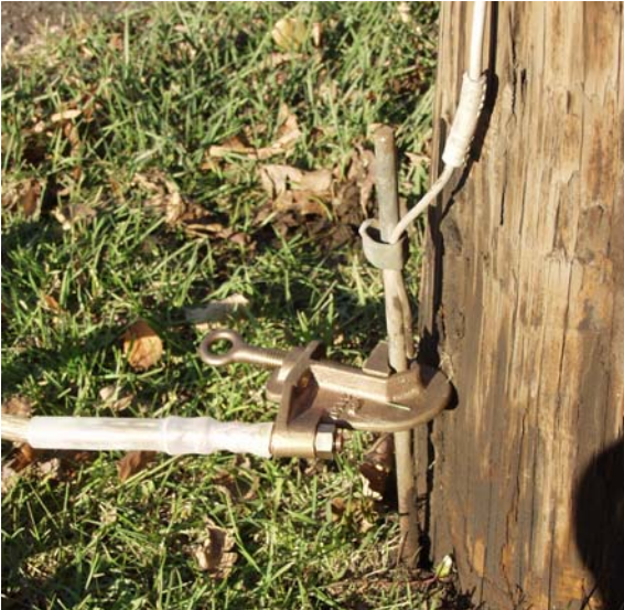
Vertical neutral of a multi-grounded neutral system
