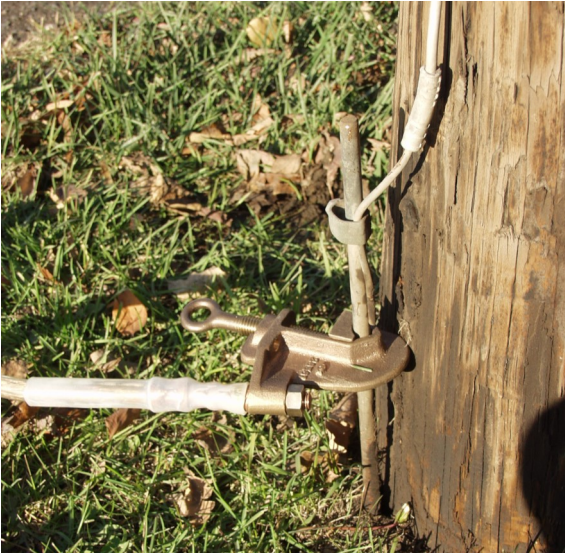
Vertical neutral of a multi-grounded neutral system
