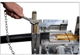
4. Clamp the sub-duct and tighten the two retaining nuts just enough to secure the duct. (Over tightening could strip the threads on the clamps)
