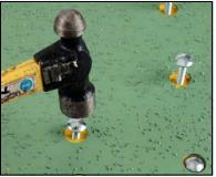
**STEP 3** Tap screws flush with a hammer sinking square under head into wood.
