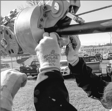
12. Place the lasher on the cable ensuring that it's centered on the strand. Close and adjust the pressure roller and secure the lifter roller.
